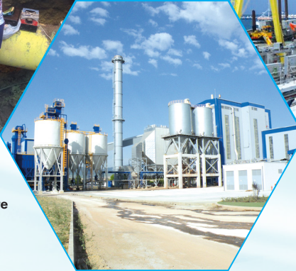
13 MW Cogeneration Facility Project
