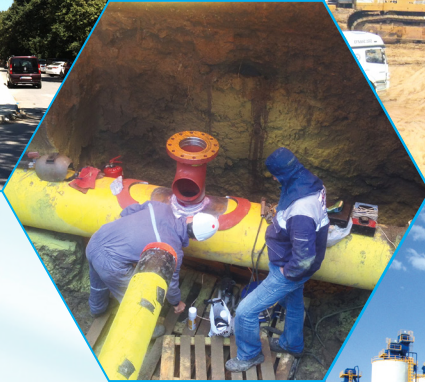
Samgaz - Selçukgaz Natural Gas Infrastructure Investment Works
